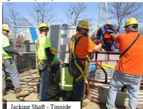
Jacking Shaft - Topside
